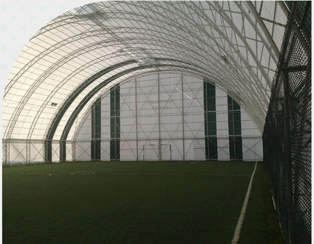
Tercan Indoor Football Field/Erzincan-Turkey
